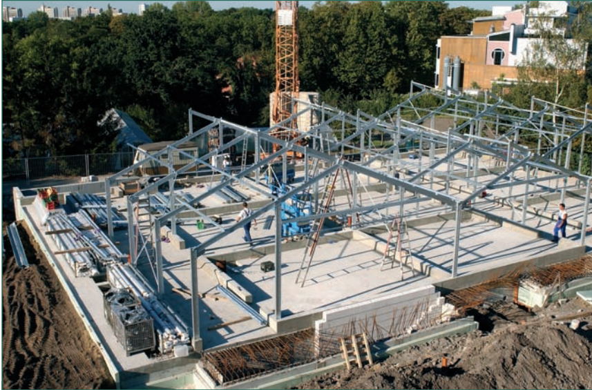
Construction of the new green houses was completed in April 2005.
